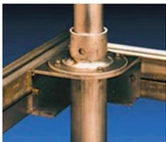
The leg supports connect to the girder structure instead of the pontoons, allowing for repeated flexing without the potential for pontoon end cap failure.
